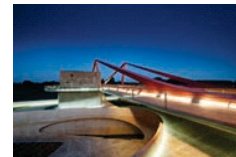
Pont enjambant le canal Albert à Vroenhoven (Riemst) © Foto_Photo: J-L Deru (Photo-Daylight)
